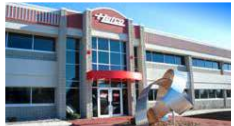
Sturgeon Bay - Manufacturing Facility 208 East Deck Street | Sturgeon Bay, WI 54235 920-743-5595
